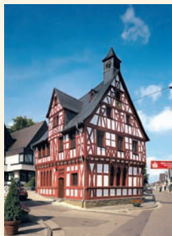
Rathaus in Rhens (M. Jeller) Rhens town hall (M. Jeller) Z. 1880/1891 (CDB 1-10-088) 1:100000 6208 (M. Jeller)
